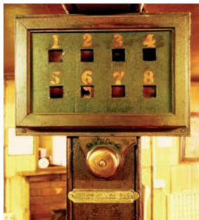
The working bell-box in the Grapes, Stranraer,
